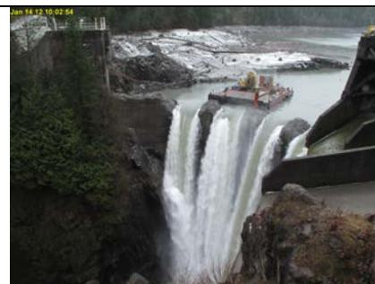
Figure 5. Removal of Glines Canyon Dam, Elwha River, WA.
