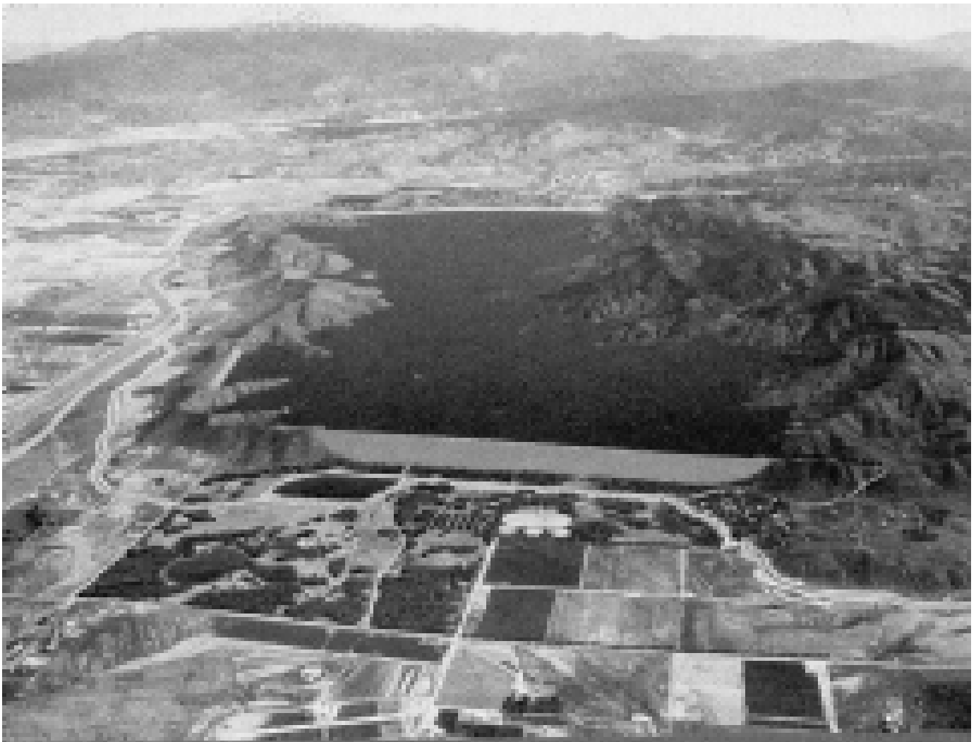
Aerial View of the partially completed Dominigoni Reservoir
