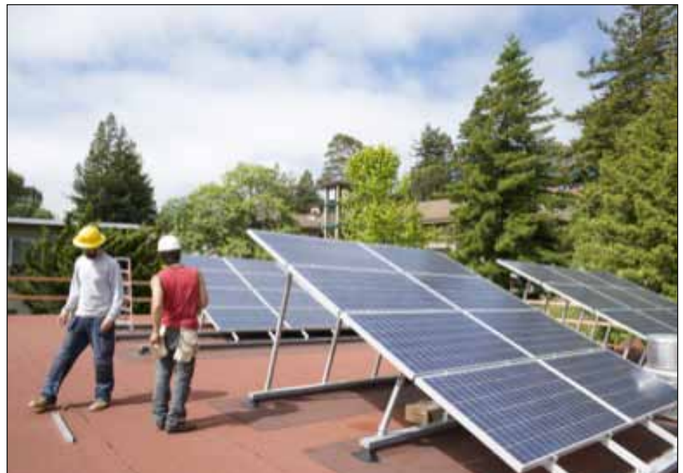
HEIF Project: Installing PV panels on the HSU Music Building.
