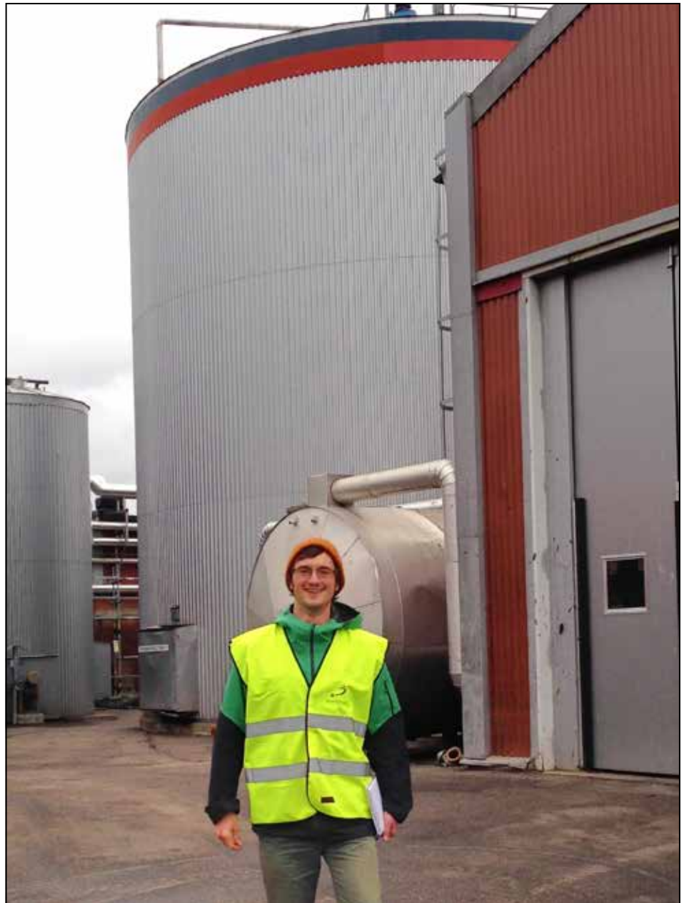
Ryan touring the centralized biogas plant in Linköping, Sweden. The plant utilizes compostable waste from residential homes to generate renewable methane to power public transportation vehicles.
