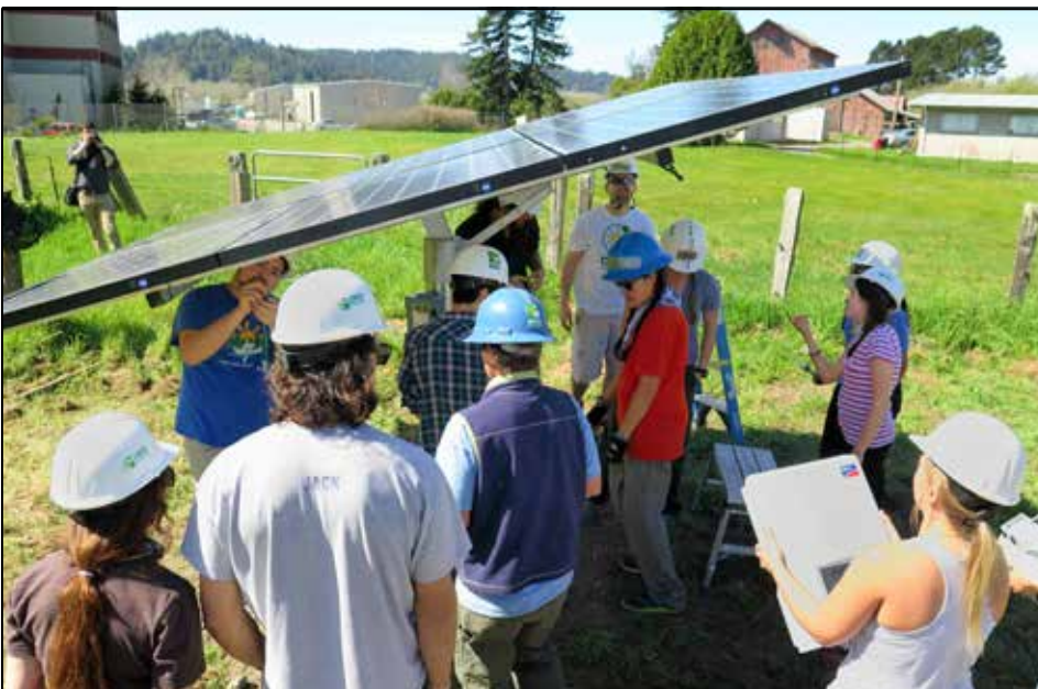
ERE students and other volunteers installing residential solar arrays in the Blue Lake Rancheria community. These systems are designed to provide 75% of a household's electricity to replace fossil energy.
