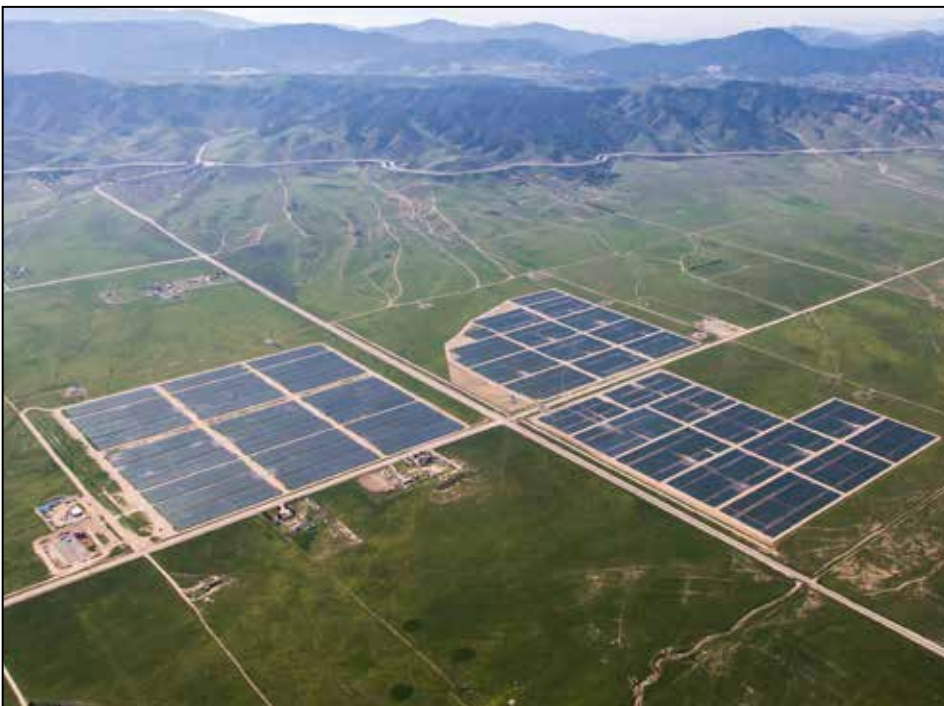
20MW West Antelope Solar Farm, Lancaster, California (2014).
