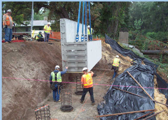
Craig Creek Bridge
