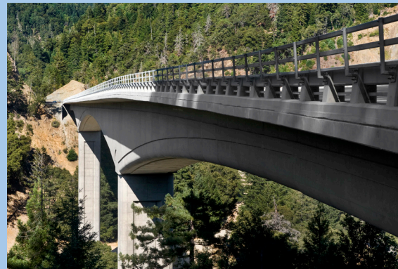
Confusion Hill Bridge
