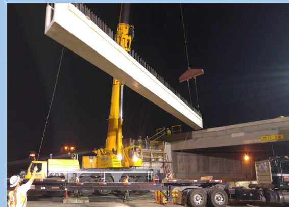
Laurel Street Overcrossing
