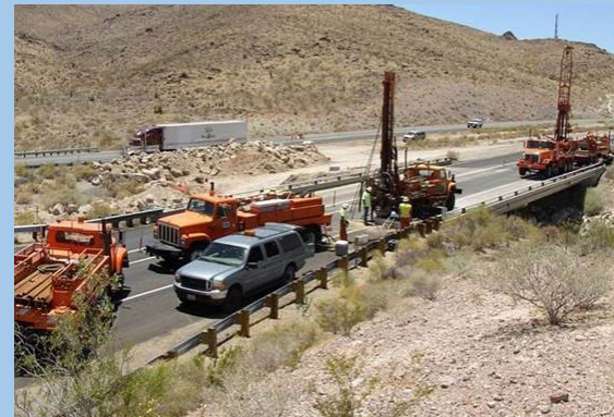
Tex Wash Bridge Replacement
