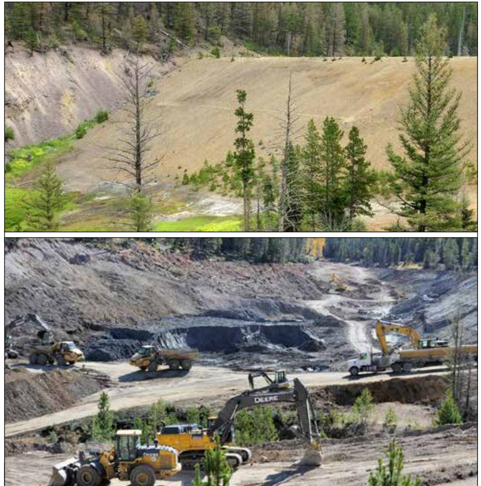
Figure 3. Mike Horse Dam, Montana. Top: Prior to removal. Bottom: During removal.
