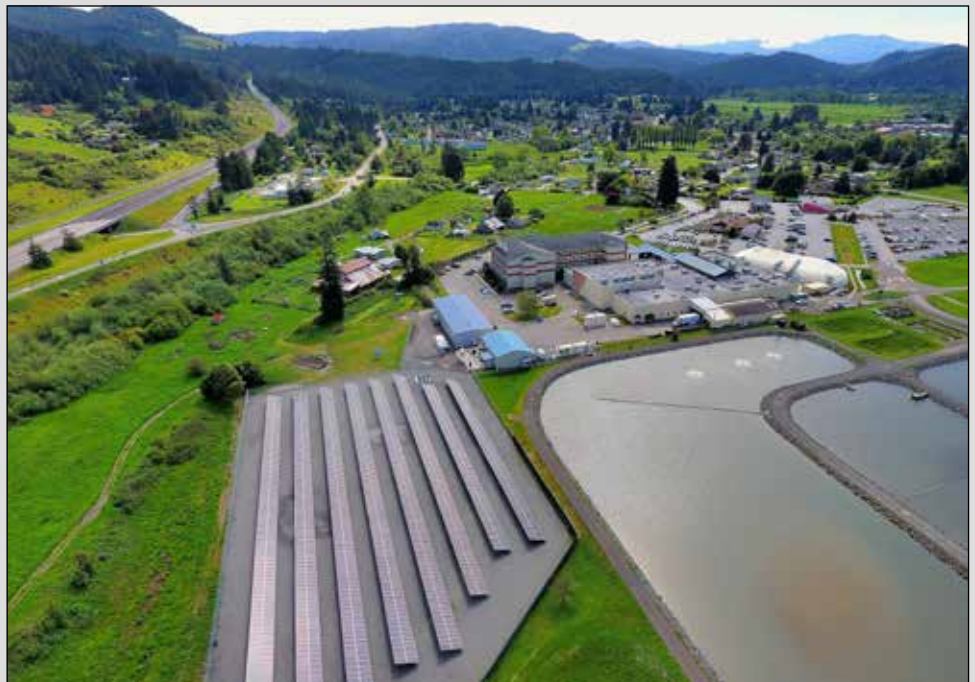
Aerial view of solar array at Blue Lake Rancheria.
