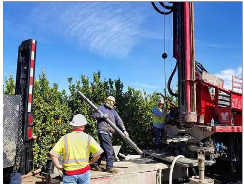
A water district drilling crew preparing to drop an anode into a well. An inspector, in the yellow safety jacket, is on the left.
