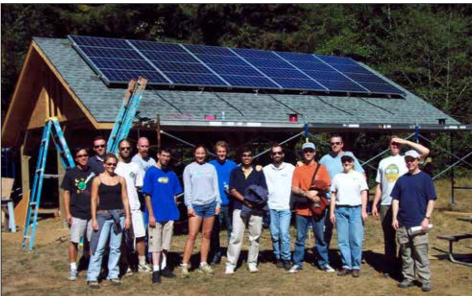
ERE students, Schatz engineers, and Redwood National Park personnel in front of the just completed PV array at the Wolf Creek Outdoor School. The project was part of the nationwide University-National Park Energy Partnership Program.
