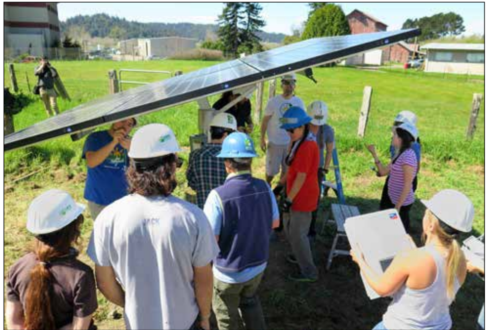
ERE students and other volunteers installing residential solar arrays in the Blue Lake Rancheria community. These systems are designed to provide 75% of a household's electricity to replace fossil energy.
