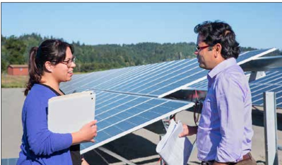
ERE undergraduate (left) and ETaP graduate student researchers on site during construction of the Blue Lake Rancheria Community Microgrid in the summer of 2016. Photo by K.J. Brown
