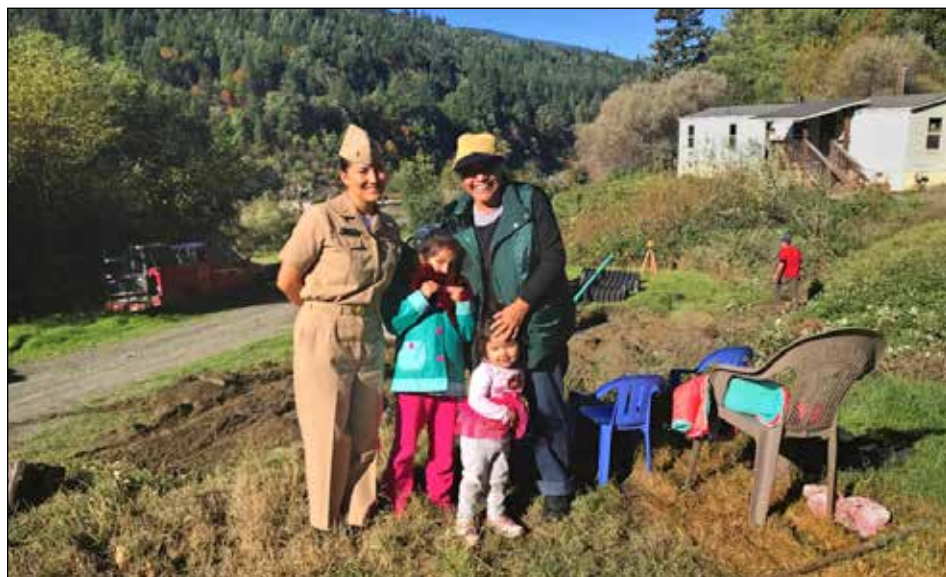
Building a leachfield with an advanced treatment system for a Yurok family in Old Village, Weitchpec on the Yurok Indian Reservation (Northeastern Humboldt County).
